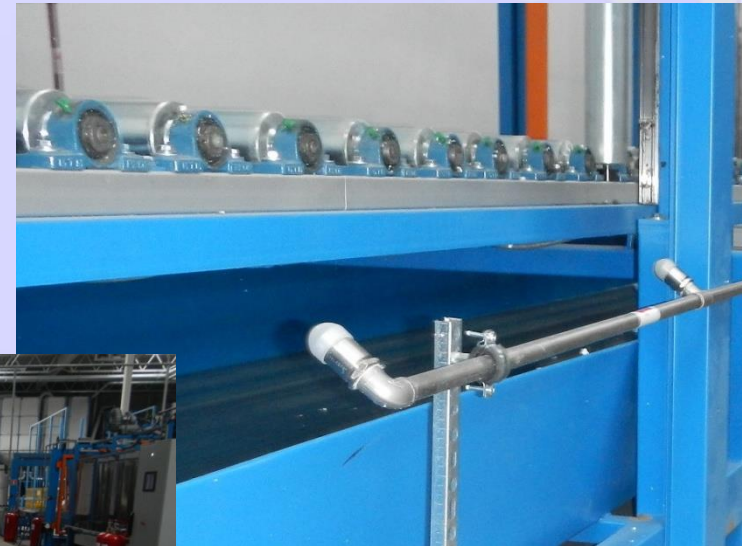
Water mist nozzle with protection cap
