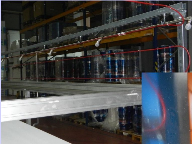
Pneumatic detection (red tube)
